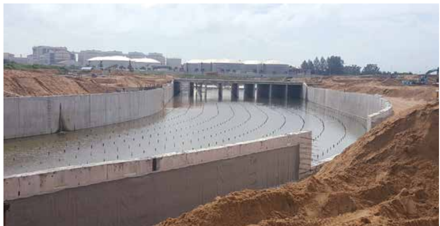
▶ Work continued apace on the Changi East development site in FY2017/18, including the construction of canals to drain water from the site.
