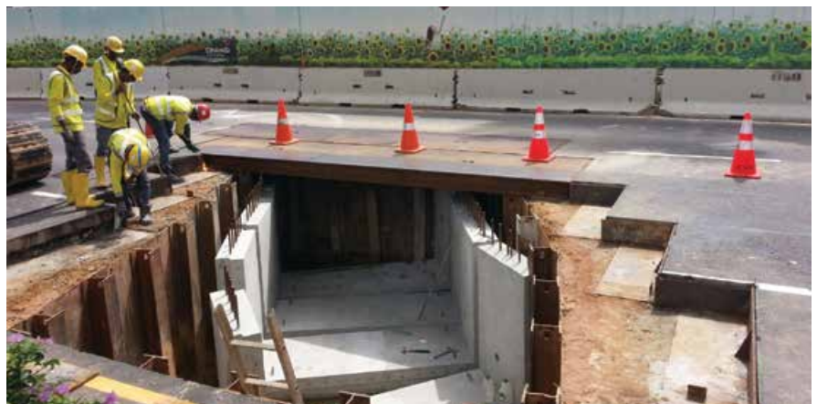
▶ The central median drain along Airport Boulevard was precast off-site to cut down on the total construction period, minimising impact to road traffic.
