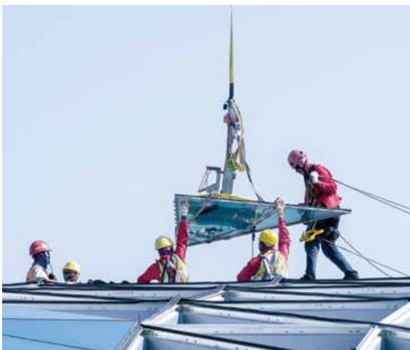
Each glass panel of the Jewel roof is carefully lifted 45m above the ground for installation.
